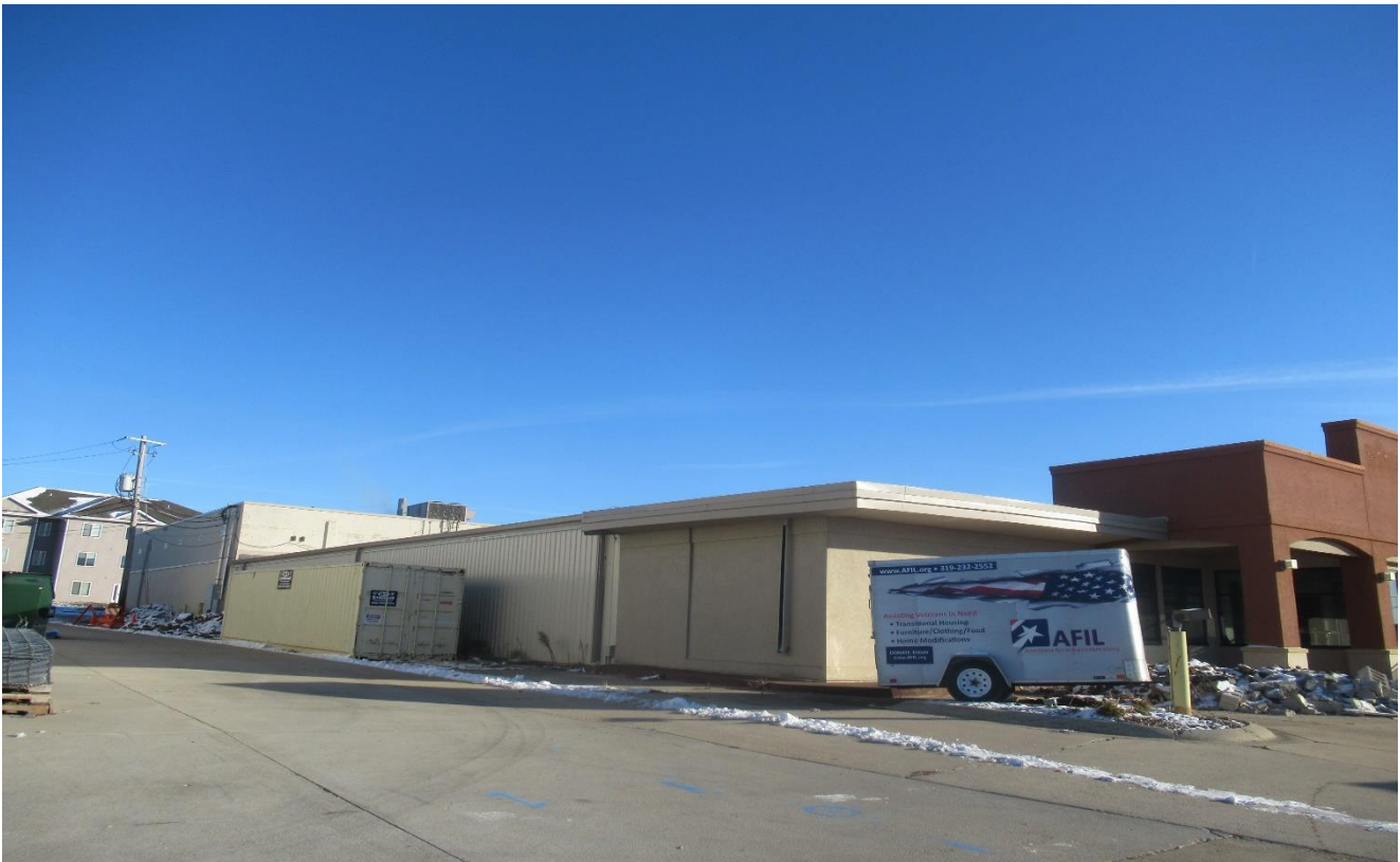
Picture 4: Looking along west side of building.
