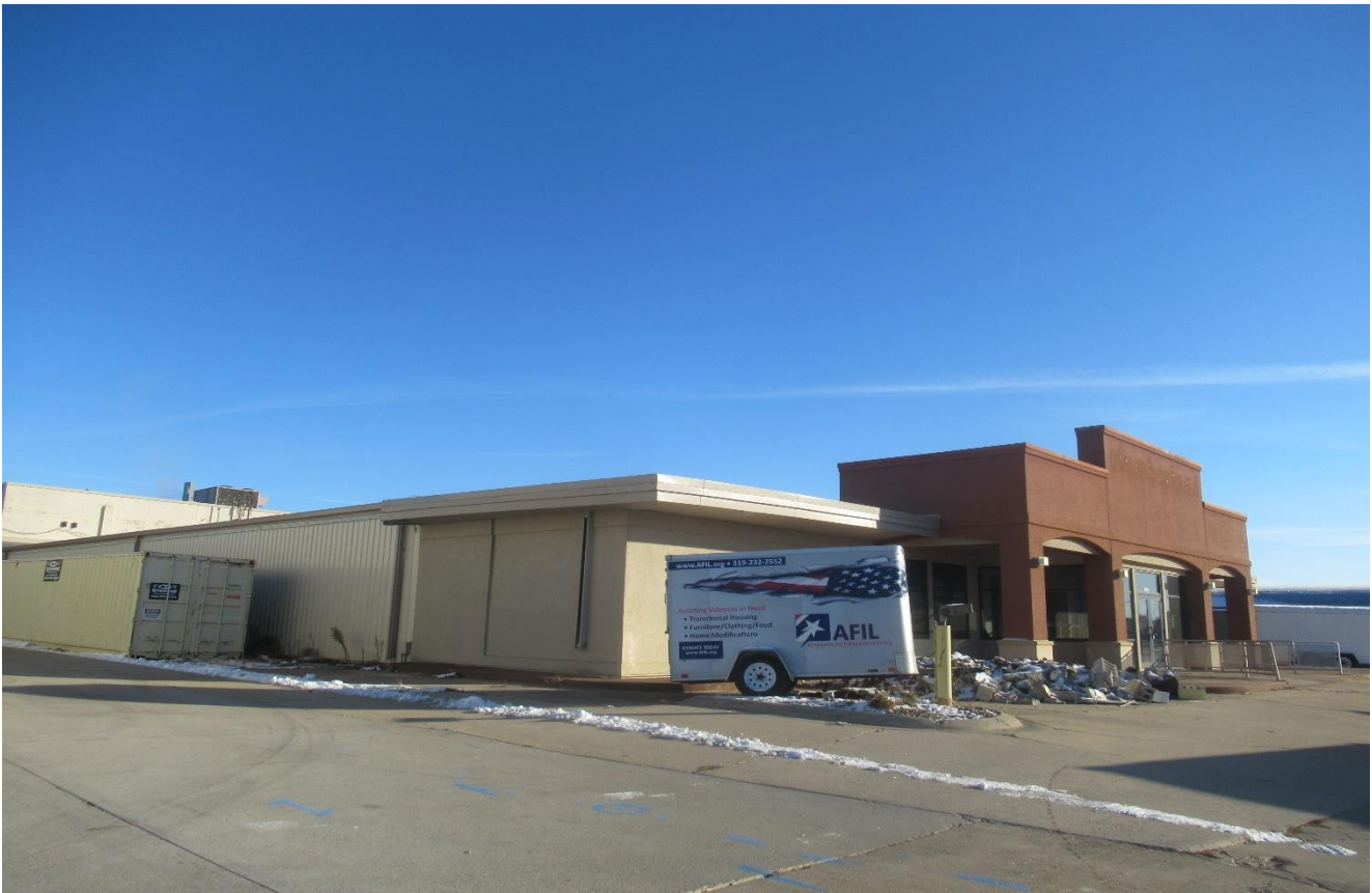
Picture 3: Front of building looking east.
