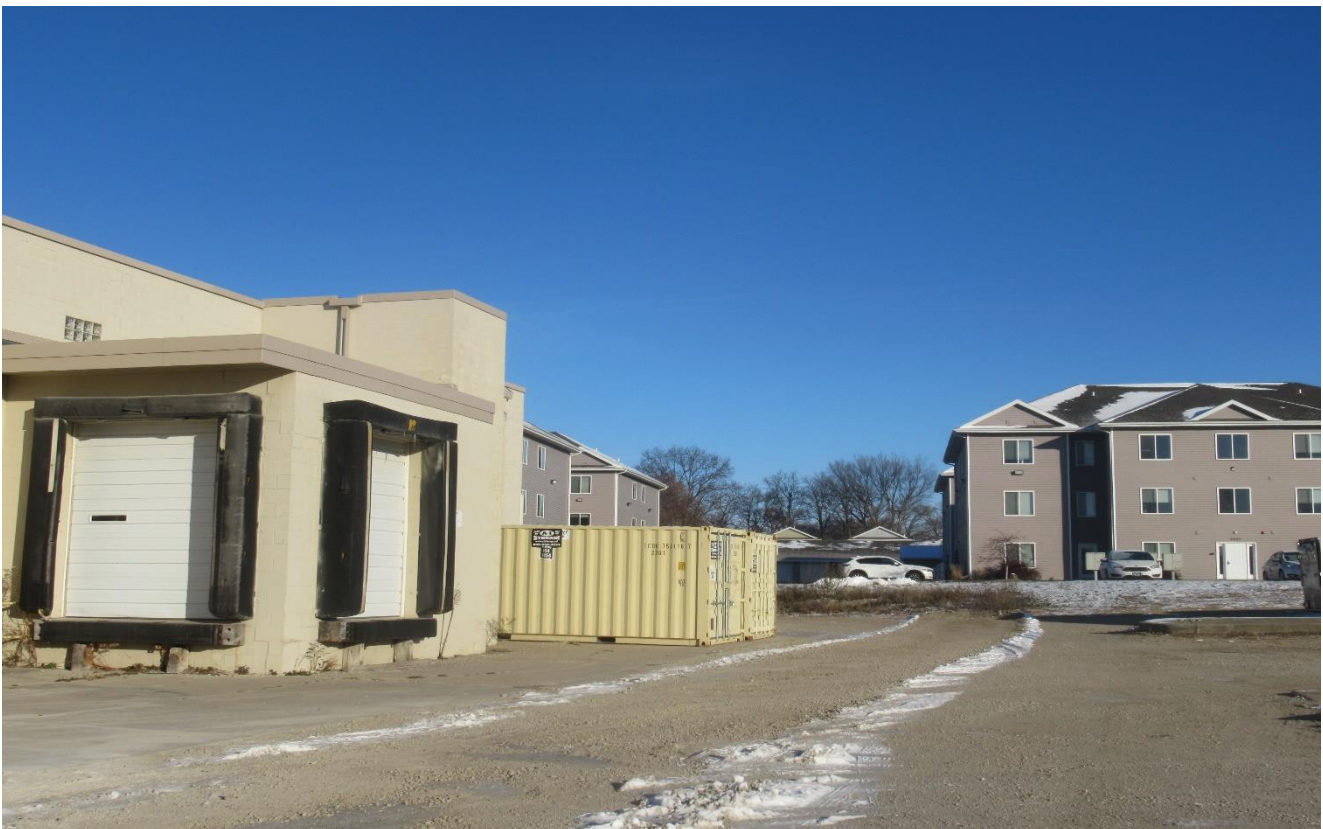
Picture 2: Rear of building looking toward apartment buildings that are behind the building in question.
