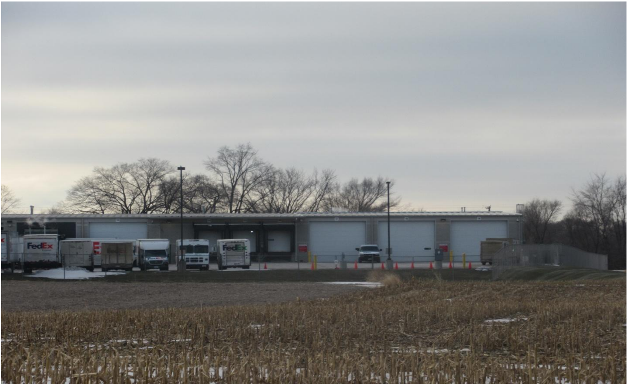
Picture 2: Looking south at the current FedEx building.
