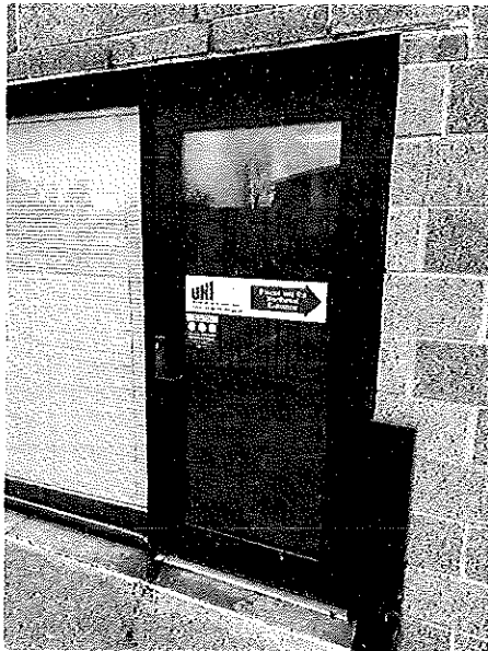
Replacement of door at UNI CUE building.
