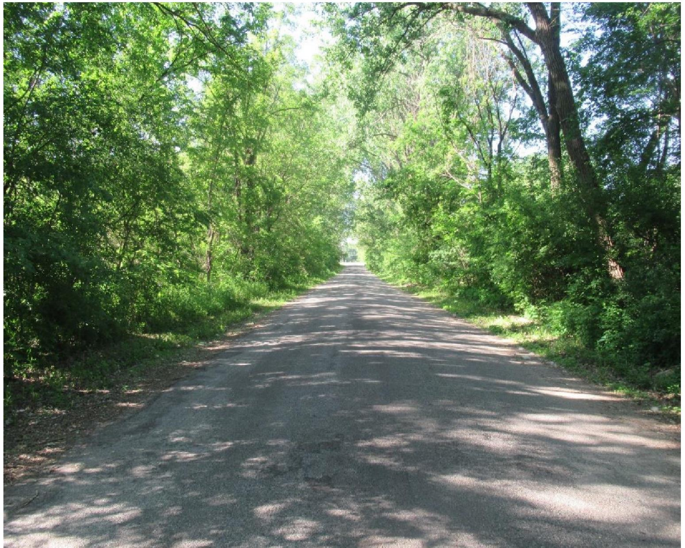
Picture 2: Looking south along East 4th Street which will be reconstructed for the project.
