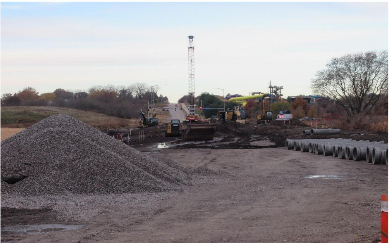
Picture 8: Current bridge work on East Shaulis just west of the rezone area.
