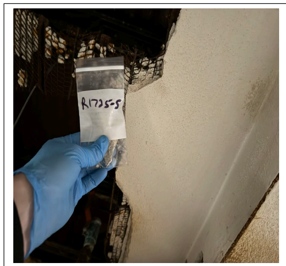
Sample R1725-5: Plaster (paint) ceiling in basement negative for asbestos from West building.
