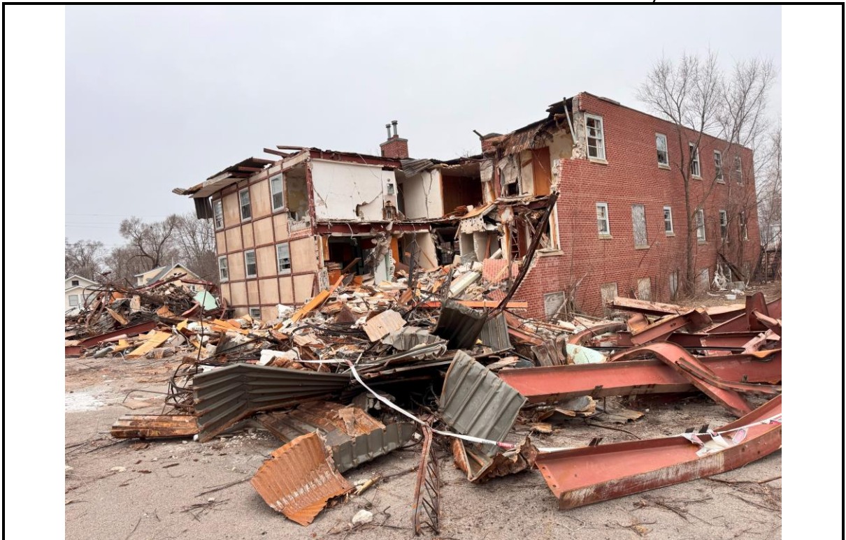
Photo 2: View looking towards the south west at the east and north elevations of the Villa.
