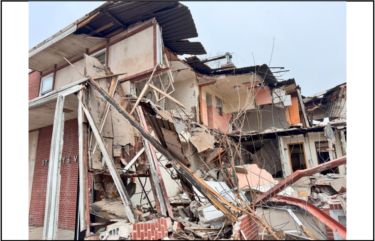
Photo 9: Photo showing the second floor/roof of the Villa.
