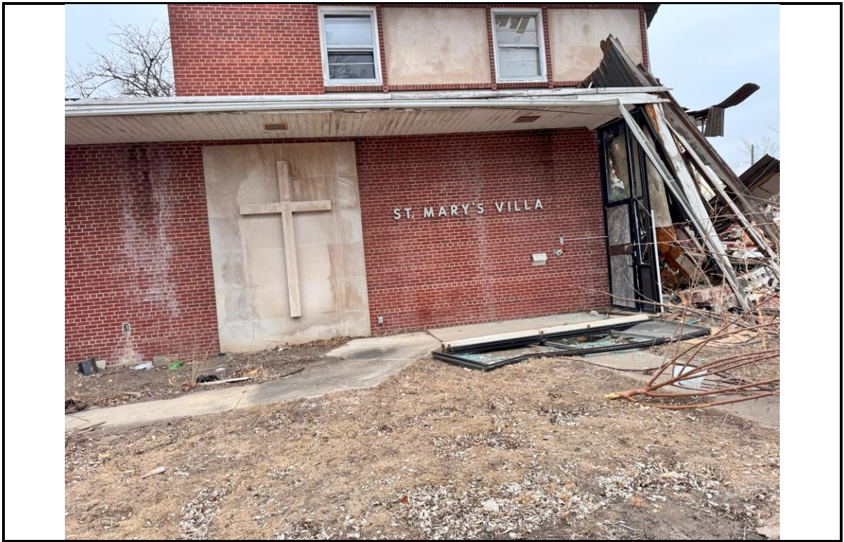
Photo 1: View of the south elevation of the former St. Mary's Villa.
