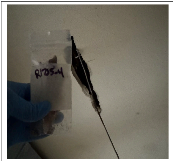
Sample R1725-4: Plaster (paint) ceiling in basement negative for asbestos from West building.
