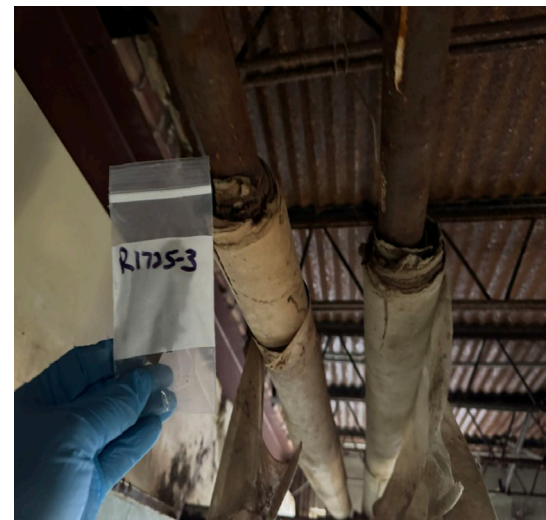
Sample R1725-3: Pipe insulation from interior of building, basement positive for asbestos. Taken from West addition not demolished yet.
