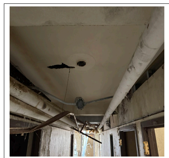
Painted plaster ceiling in basement of West building negative for asbestos.
