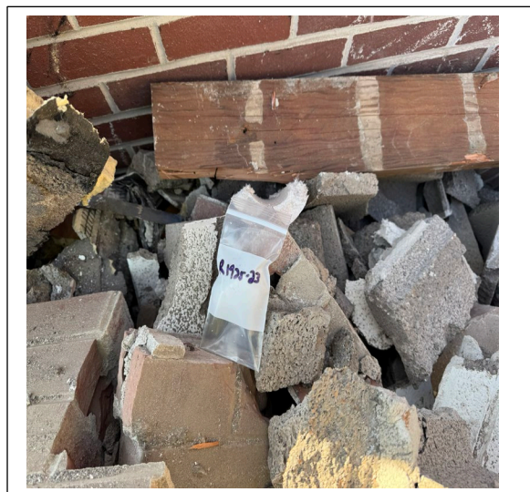
Sample R1925-23: Mag pipe debris from SW addition of larger building positive for asbestos.
