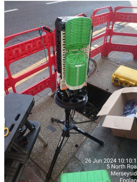
Document each Fiber in a splice tray, the direction, the use, the customer and if in use or not or even if spliced.
