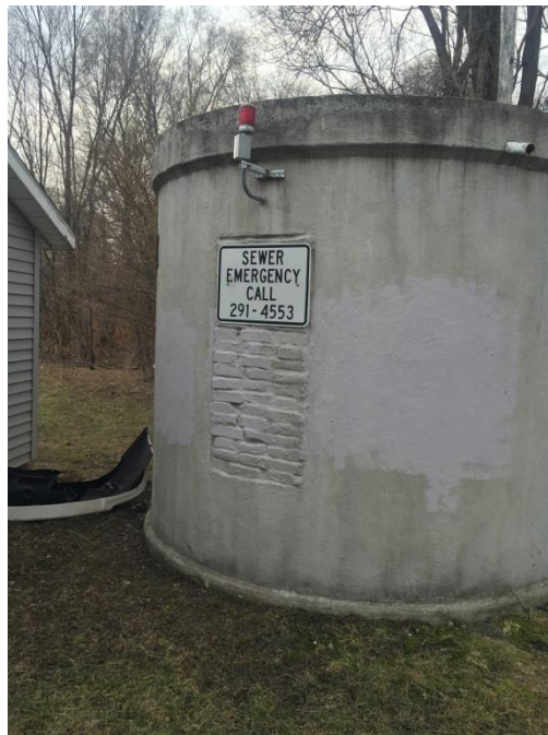
Picture D5: Patched Window and Concrete Coating
