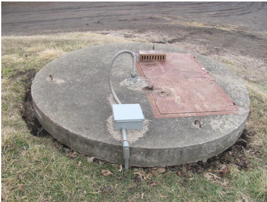
Picture CC6: Wet Well Exterior
