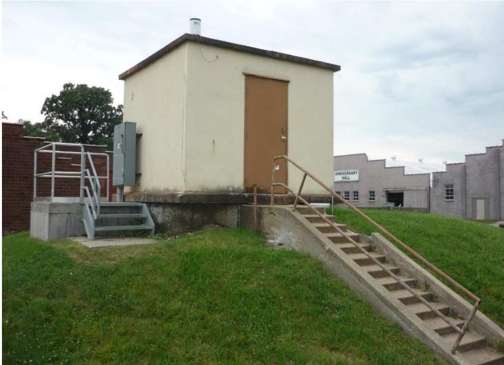
FIGURE 3: Existing Cattle Congress Lift Station
