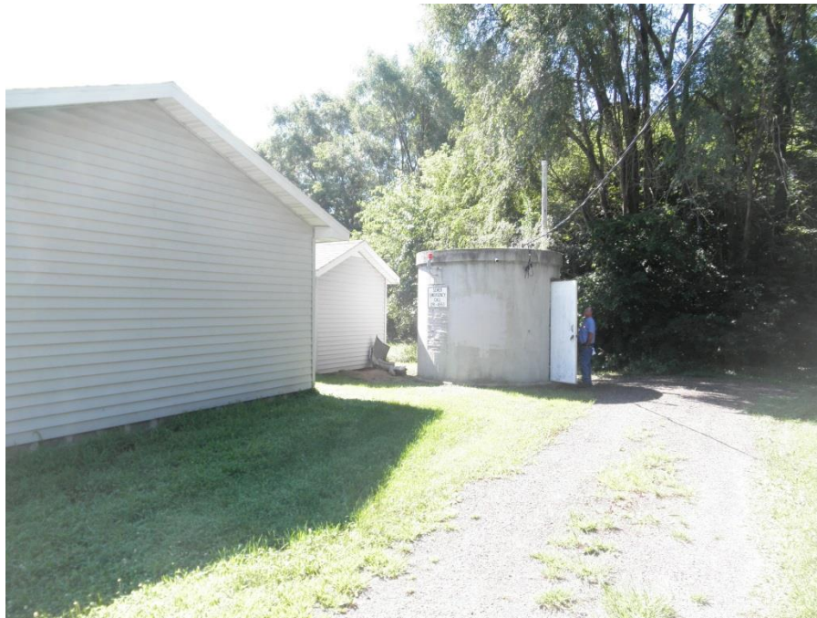
Picture D1: Douglas Street Lift Station; Note Close Proximity of Residential Structures
