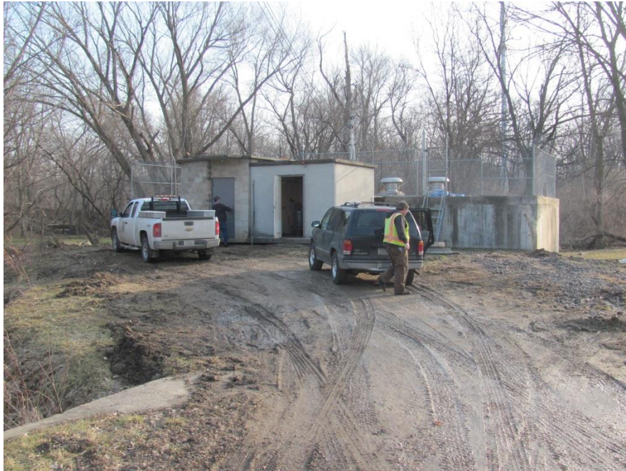
Picture NH1: North Hackett Road Lift Station
